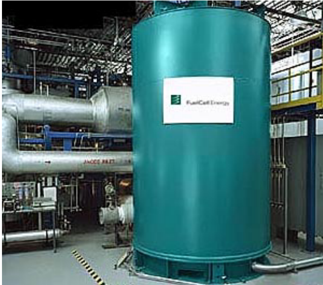
US DOE's 250 kilowatt- Direct Fuel Cell
